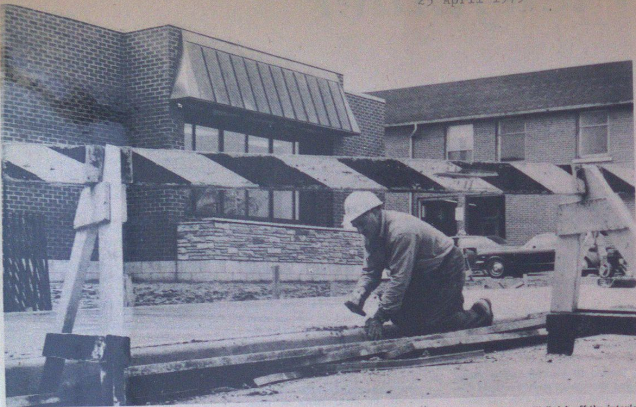
Tillsonburg and area residents can finally get a good look at what has been going on behind the fences over the winter, as the boarding around the new Tillsonburg Public Library came down this week. Outside finishing touches, like the front sidewalk, are
